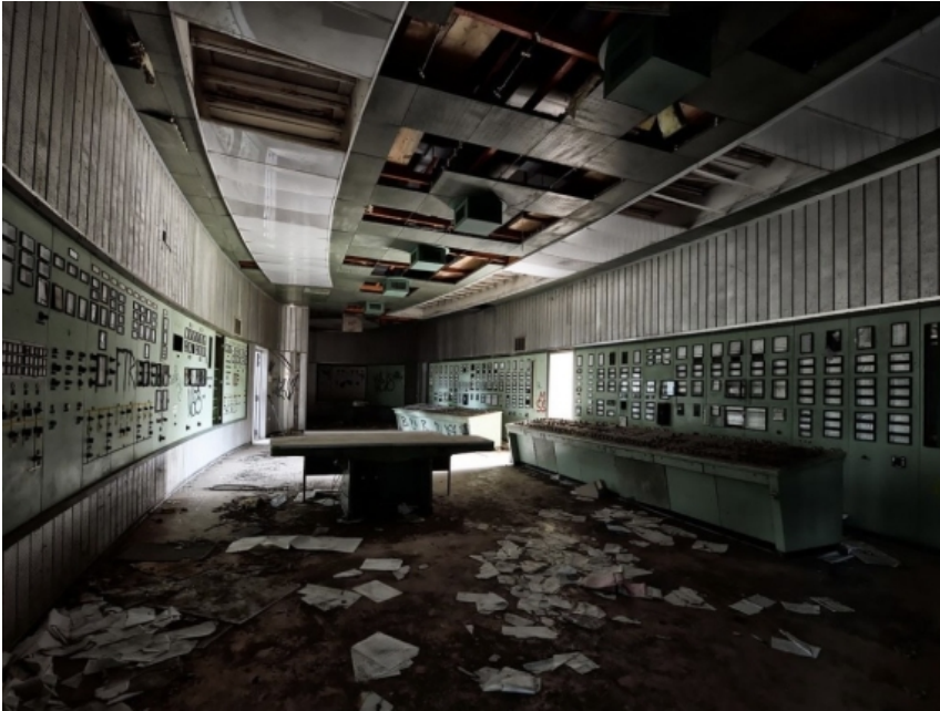
The interiors of the old power station
